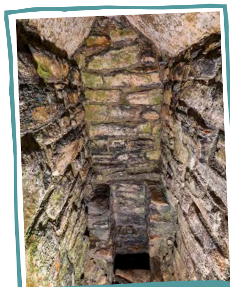
The inside of the latrine and its chute in the east curtain wall at Richmond Castle.
