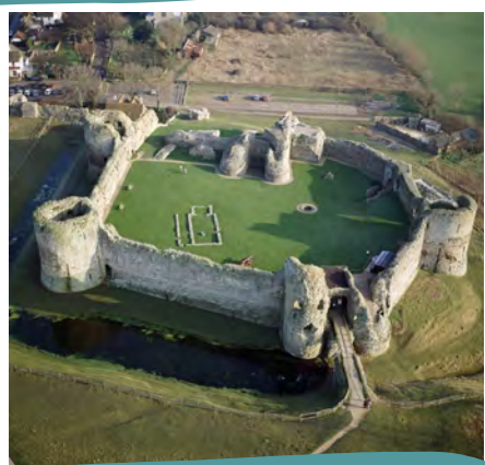
An aerial photo of the inner bailey at Pevensey Castle.
