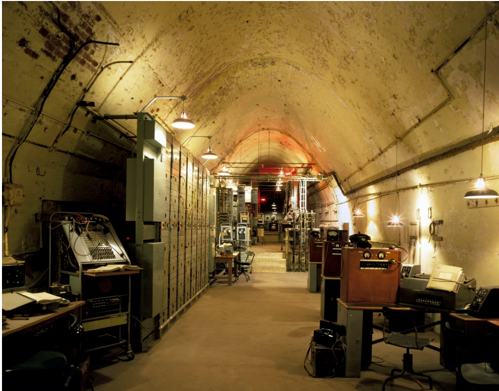
Figure 1. The Repeater Station in the Secret Wartime Tunnels at Dover Castle.
